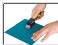
step 1: make grid cutting on surface
